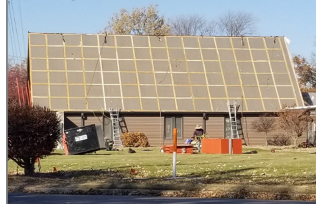
Completed Insulation
