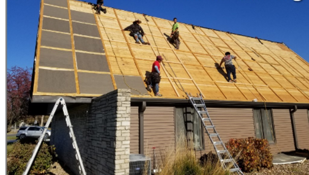
Install Foam Insulation For Sound & Thermal Management
