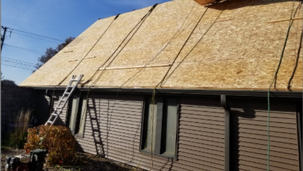
Secure Insulation & Cover with OSB
