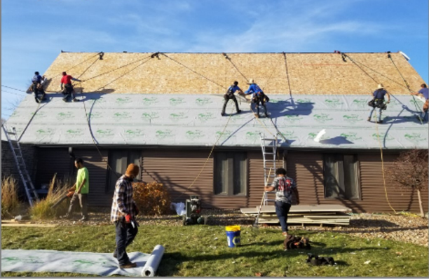
Secure Insulation & Cover with OSB
